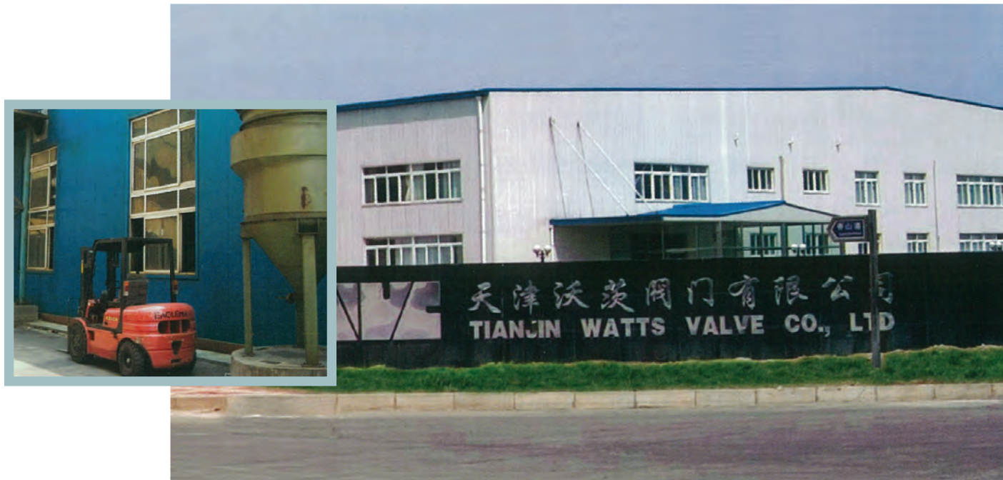
Watts opened its new state-of-the-art 125,000-square-foot Tianjin Watts Valve Company plant in the fall of 2003 to machine the castings from the Tianjin Watts Bronze Foundry. The Tianjin Watts Bronze Foundry, with a capacity to produce more than 200 tons of finished castings per month, was an outgrowth of Tim Horne's vision.
