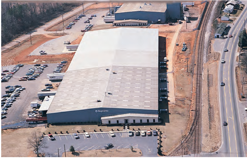
Watts built a new manufacturing plant in Spindale, North Carolina. The North Carolina plant came into its own as the center for high-volume plumbing and heating products, freeing up some space and personnel at the Franklin, New Hampshire, plant, which could then focus on industrial products.
