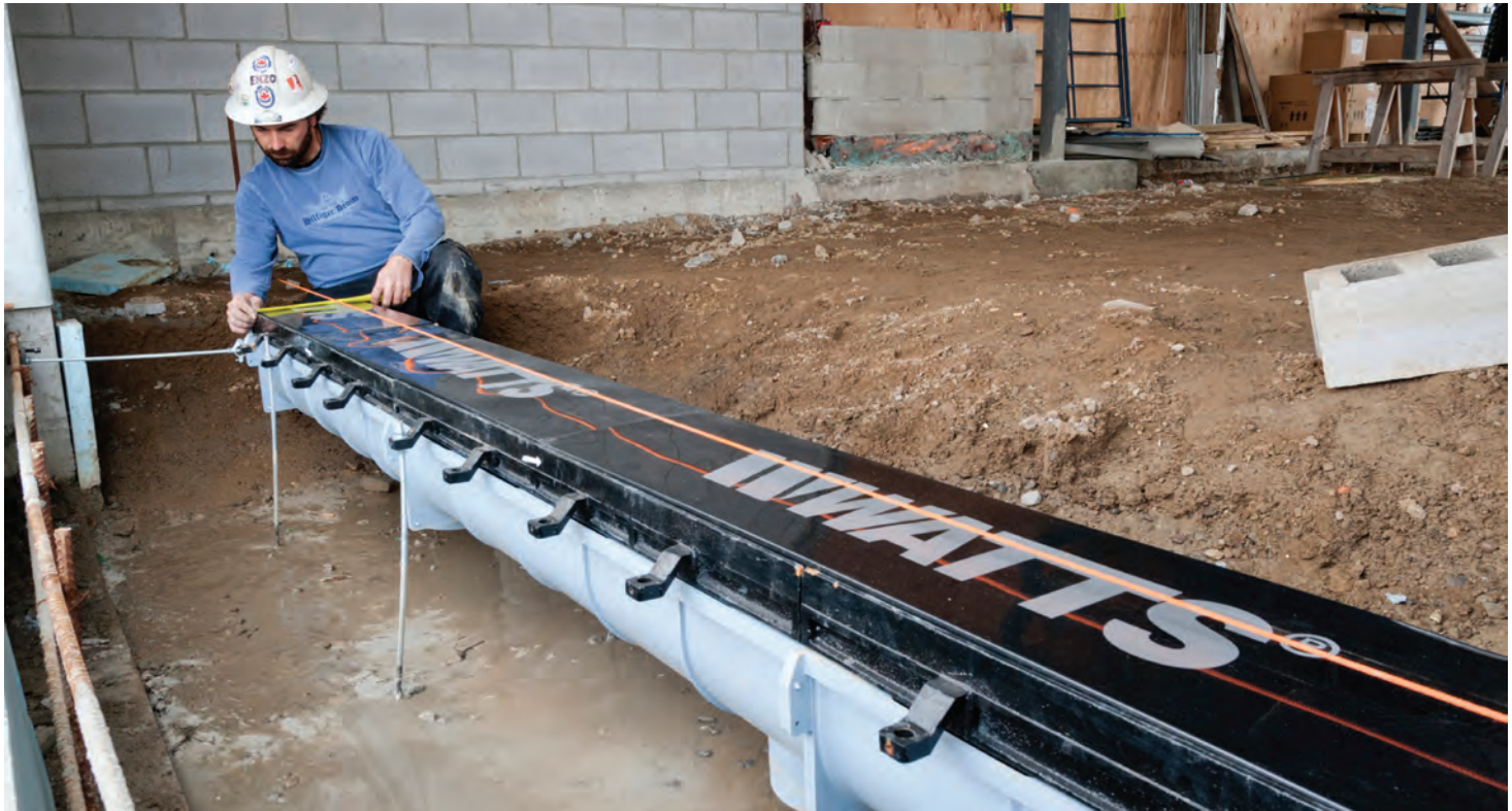
A Watts Dead Level® trench drain installation.
