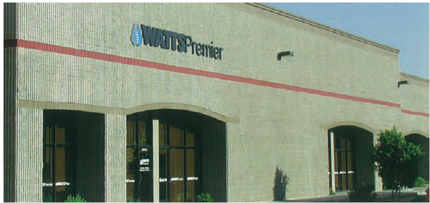
The acquisition of Premier Water Systems ushered Watts into the RO technology for purifying water.
