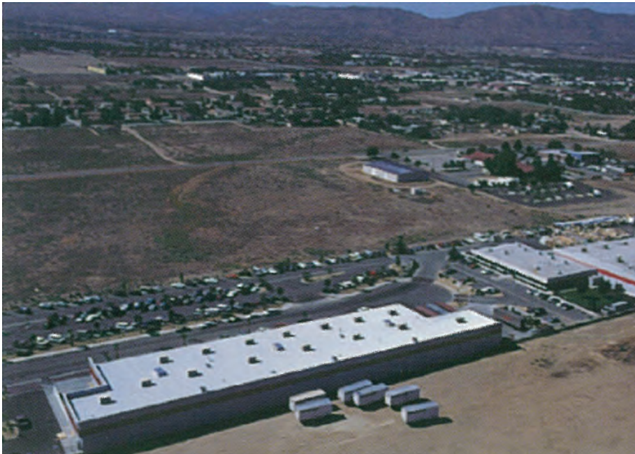
The large, highly automated Anderson-Barrows plant in Palmdale, California, produces high volumes of hose connectors and brass fittings for the retail-oriented DIY market.
