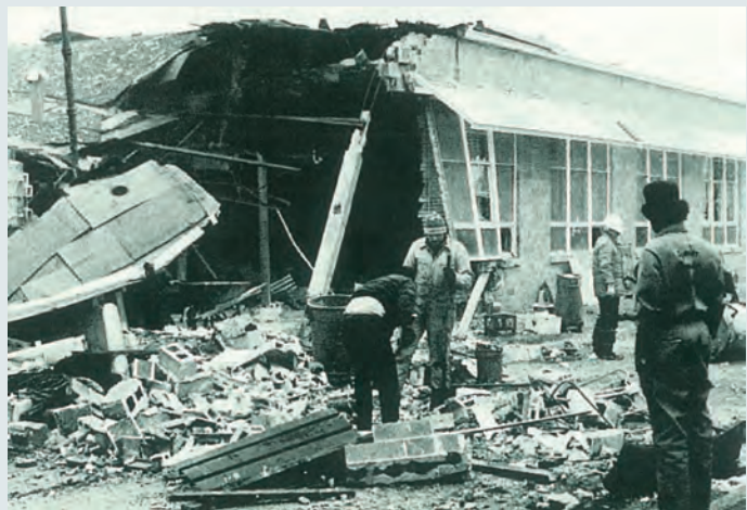
George Horne also constructed dramatic presentations of mounting pressure and its consequent explosions, displaying the necessity for T&P valves.
