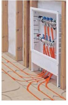
for a lower temperature heat input to achieve a comfortable temperature. The German Heating Industry Association estimates that with radiant floor heating, room temperature can be reduced by 2°C and provide the same comfort level.
