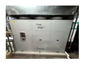
hot water. CO2's official refrigerant code is R744 and is non-toxic, non-flammable, has an Ozone Depletion Potential (ODP) of zero, and a low GWP.
